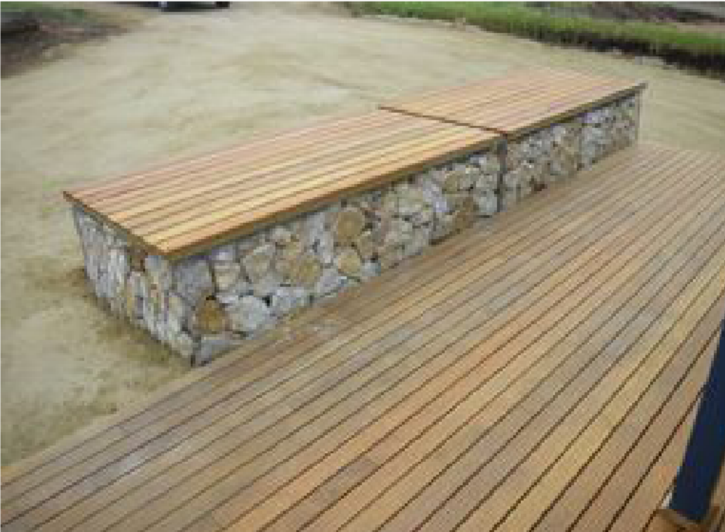
INTERGRATED WALL AND SEATING
