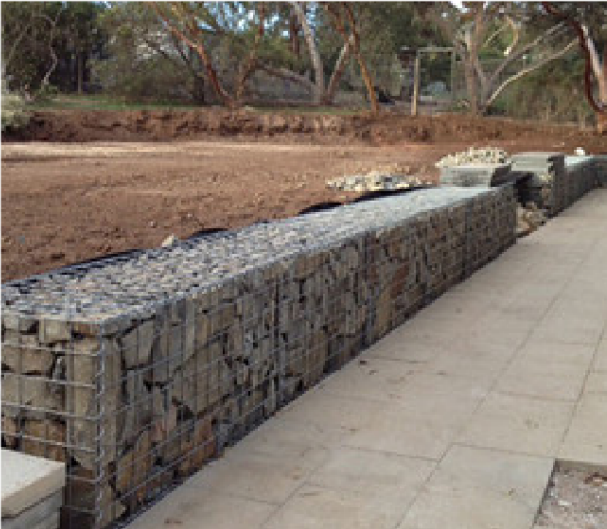
BABION WALL STRUCTURES
