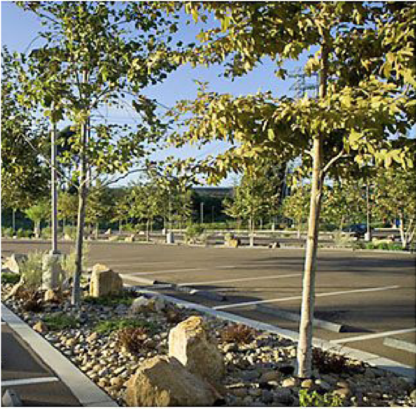
RAIN GARDENS WITHIN AND ADJACENT CARPARKING AREAS UNDERTAKING BIO FILTRATION OF STORMWATER RUNOFF
